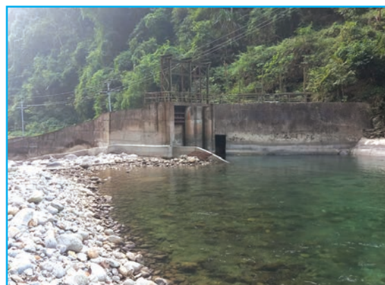
Intake and gravel trap
