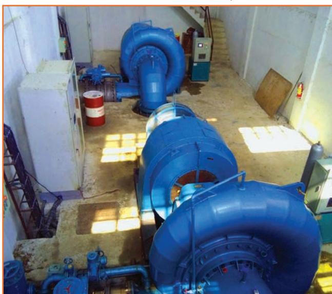
Powerhouse machine floor with turbine and generator
